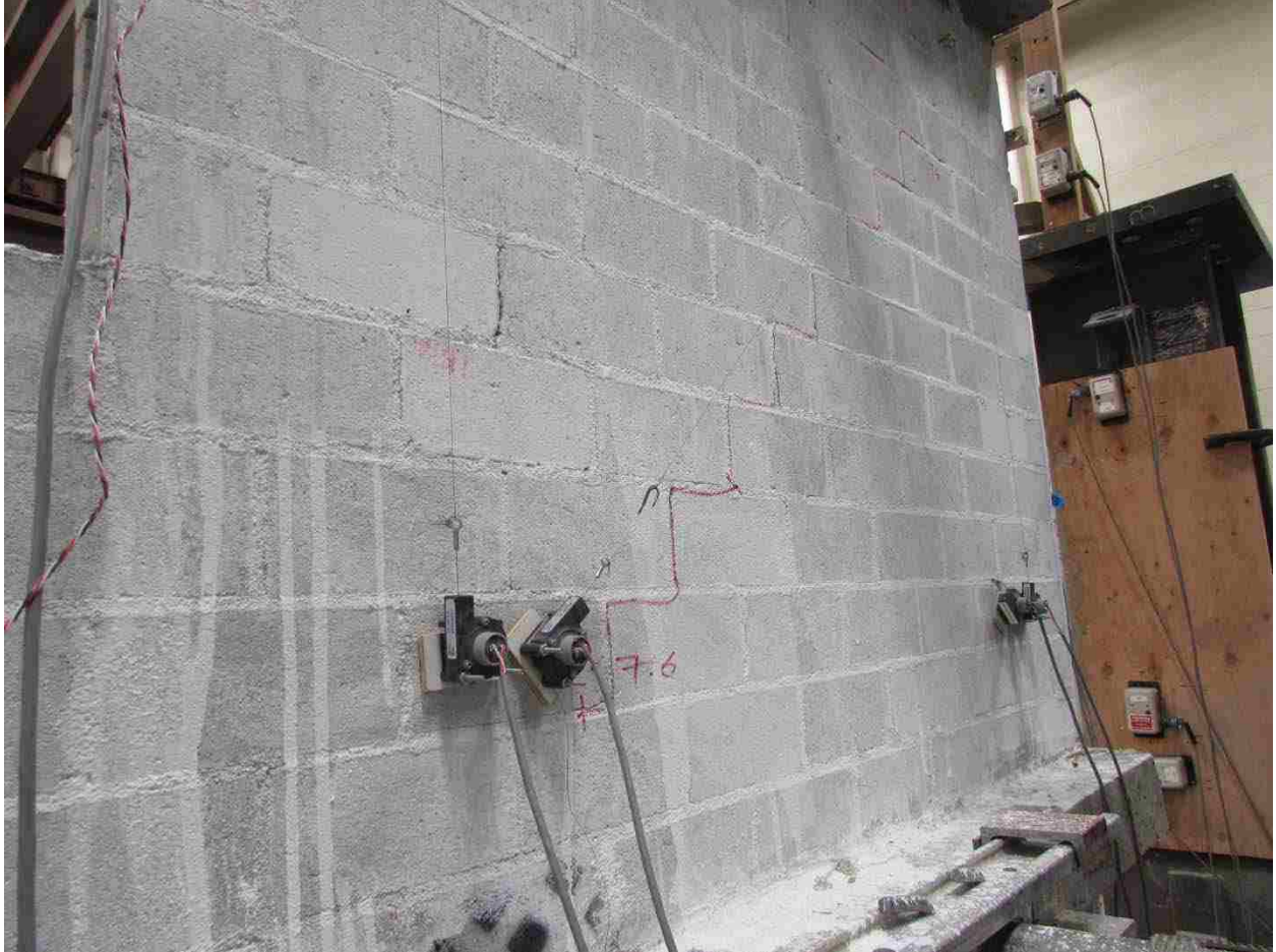
Figure C-6: Enlarged view of 3 rd story cracks in pull regime
