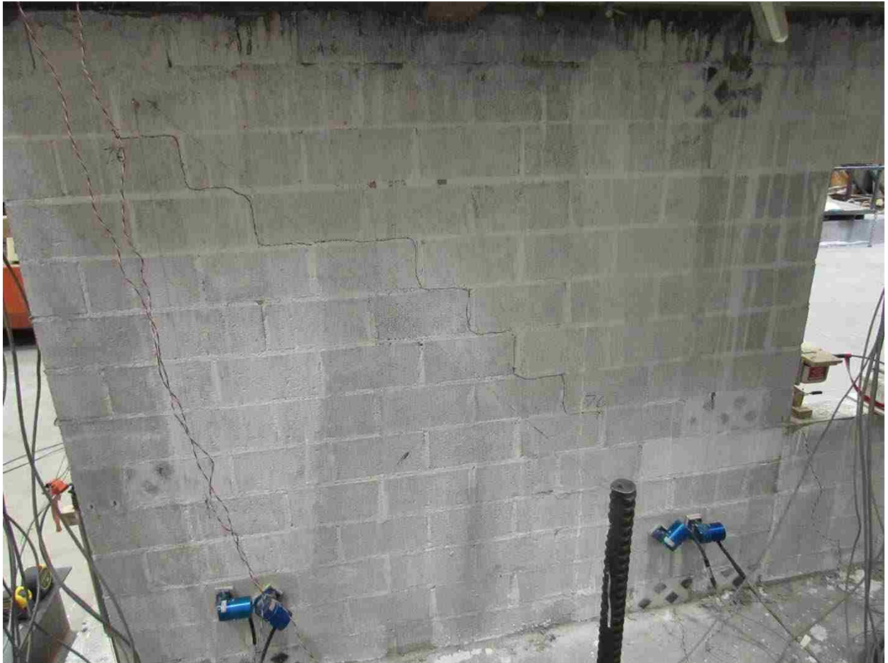
Figure C-1: Enlarged view of 1 st story cracks in push regime
